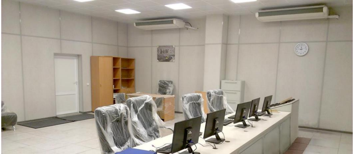
Fig.3. BF Central Control Room
